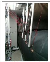
Figure 22: The three hanging overinflation switch mechanisms are shown with a half-filled bladder. The liquefier manifold is against the left wall.
