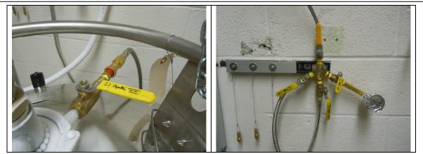
Figure 15: (a) The dewar blow-off exhaust port vents through a 2 PSI check valve and a Swagelok quick connect. (b) The mobile dewars vent into the dewar helium blow-off capture manifold. This manifold attaches directly to the liquefier 150L dewar reservoir.
