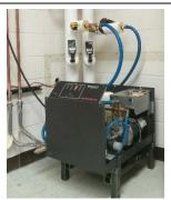
Figure 17: A Coherent LaserPure 20 chiller supplies chilled water to the Cryomech LHeP22. It is a closed-loop circulator chiller with a water pump and heat exchanger. The physics building supplied chilled water cools the heat exchanger.
