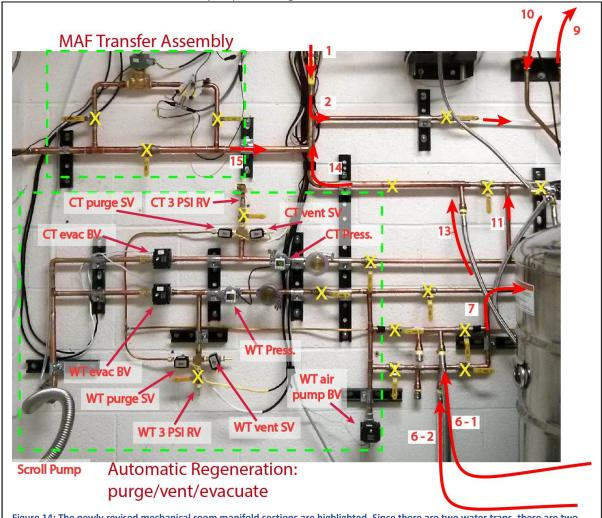
Figure 14: The newly revised mechanical room manifold sections are highlighted. Since there are two water traps, there are two junctions, one at 6-1 from water trap #1 and the other at 6-2 from water trap #2. The helium continues through the system as described earlier, steps 7-14. One trap can be isolated from the system and be regenerated while the other trap is in service.
