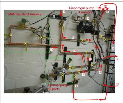
Figure 10: The main sections of the liquefier room manifold are shown. The red arrows and sequential numbers show the helium gas flow from the bladder through the system under normal run-time conditions, and the yellow x's demarcate manual valves.
